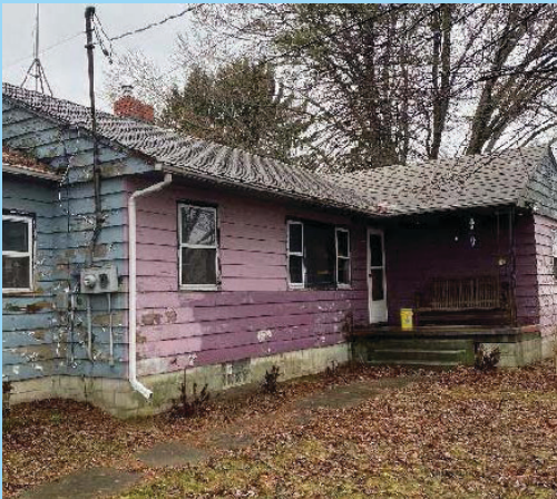
Before Lead Rehabilitation
