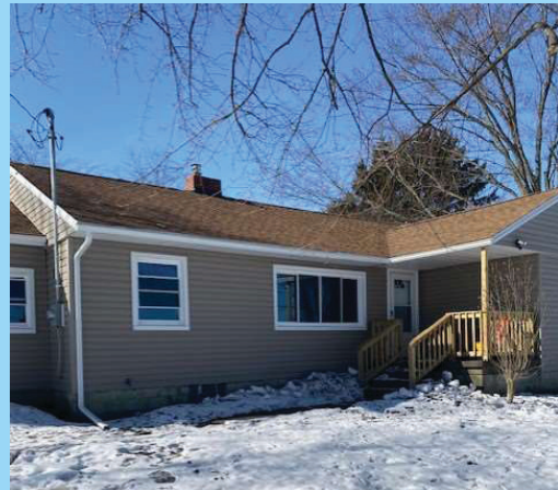
After Lead Rehabilitation
